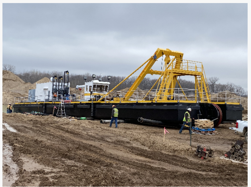
The new electric powered Cutter Suction Dredge being assembled at Legacy Materials in Booneville, IA
